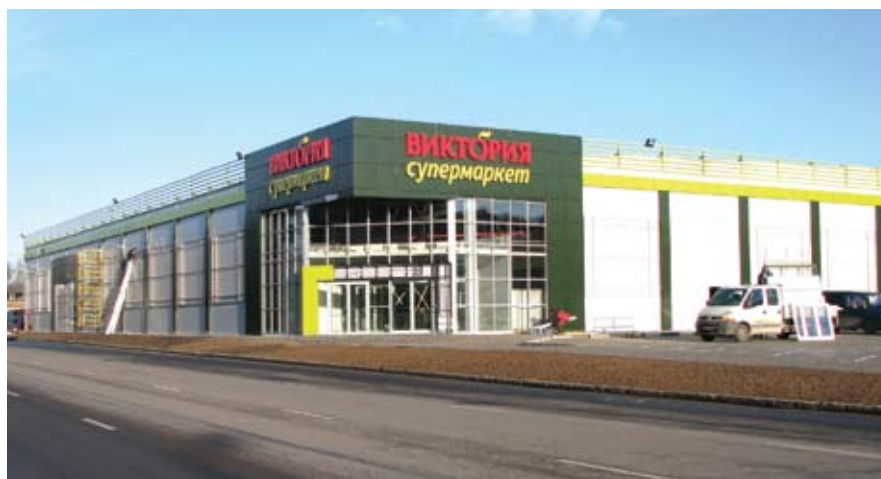
The construction of the supermarket in Kaliningrad (Russia).
