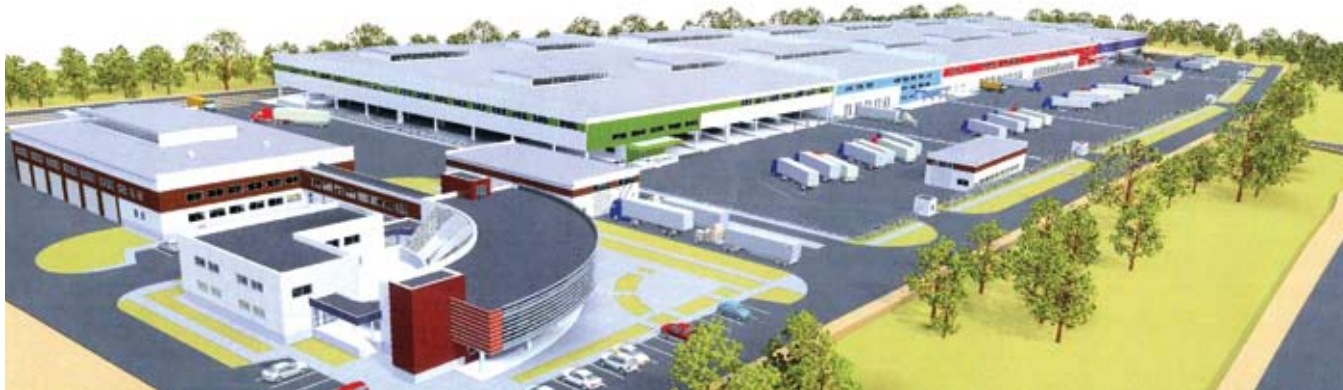
The decoy of the warehouse in Yekaterinburg (Russia).
