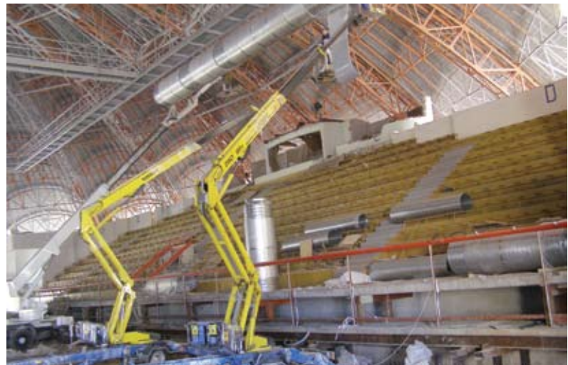
The reconstruction works of an ice arena in Elektrenai (Lithuania). An installation of ventilation equipment.
